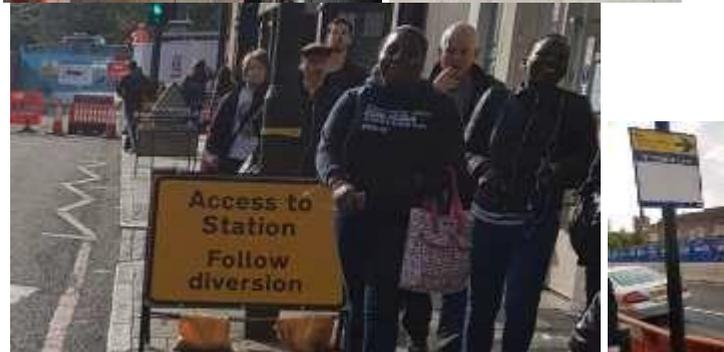
Signage clutter observed around entire works footprint causing obstructions to pedestrians and cyclists.
