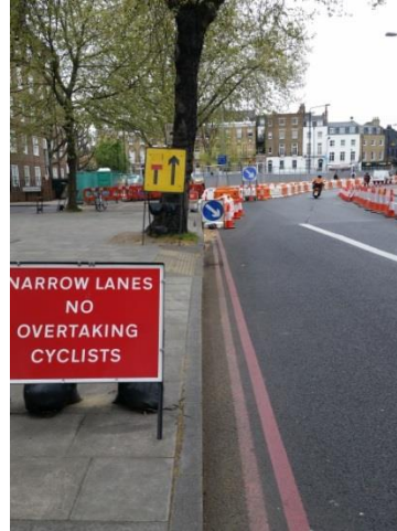
Distance to hazard unclear in traffic conditions. Short transition from 2lane to 1lane over length of crossing's zig zags
