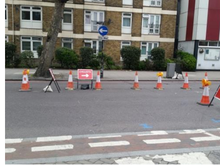
3. St Georges Road – counter intuitive sign for a temporary “two way cycle track”
