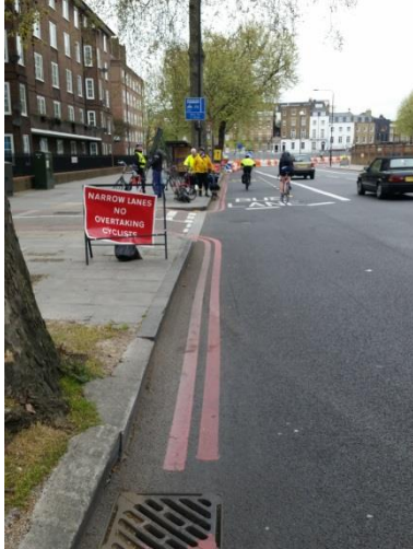
5/Kennington Road - poor signage
