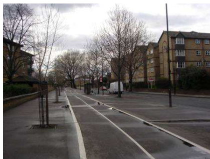
Separated on-pavement cycle lanes
